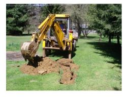
To prepare a soil profile examination, the permit Applicant is responsible to have a suitable sized backhoe or excavator on site to dig the test pit(s). The size of the pit will be a maximum of 8 feet deep, and wide enough and tapered on one end so the SEO can get in and out. It is best to schedule the backhoe so that all interested parties and the SEO can be at the site at the same time.
